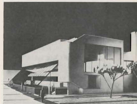
The new life sciences building now under construction on the Forsyth side of campus will provide badly needed biological research and library facilities.
