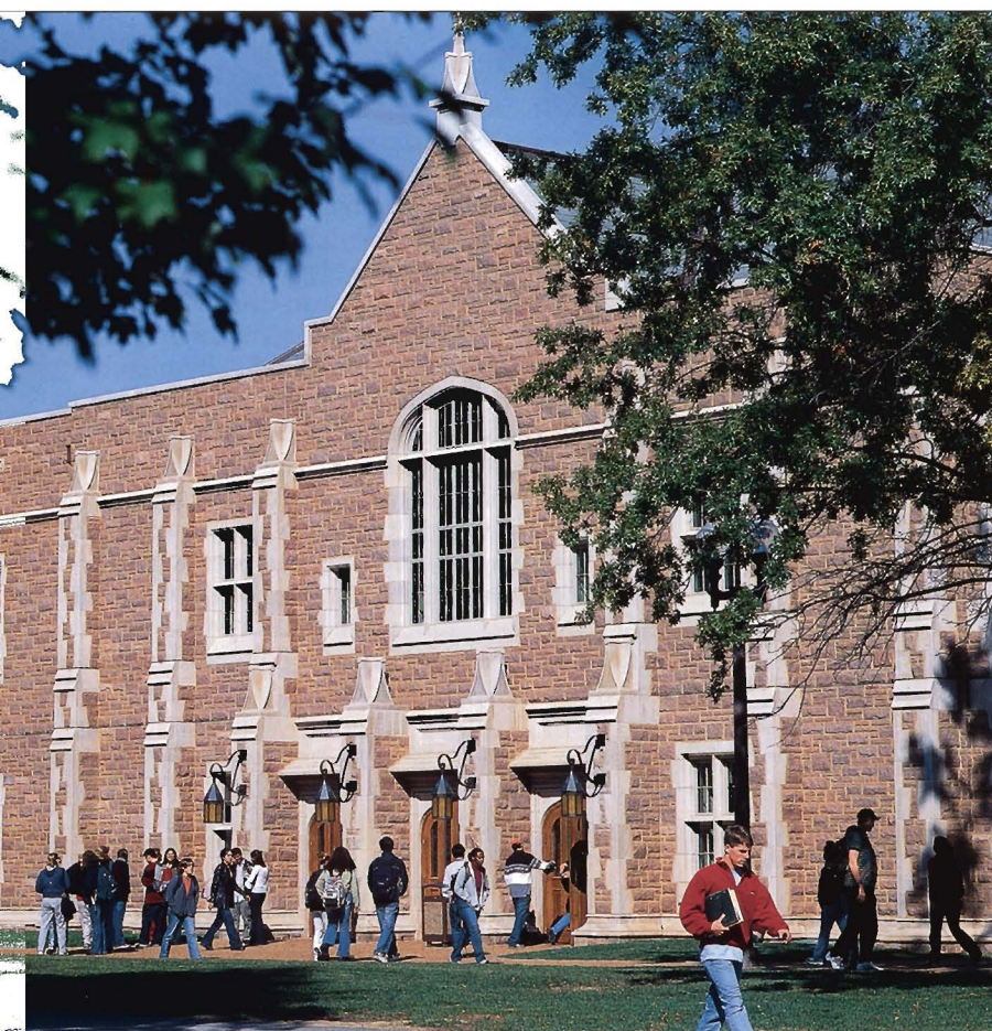
The recently completed Arts & Sciences Laboratory Science Building is the new home for the Department of Chemistry.
